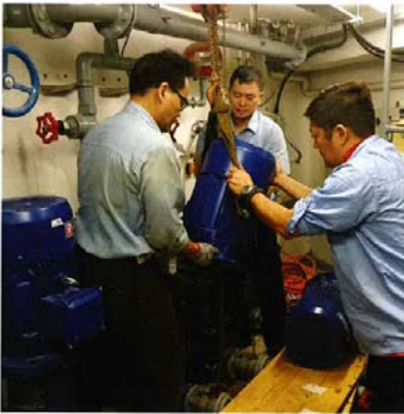
Dismantling of the motor for flushing water up-feed pump-1
